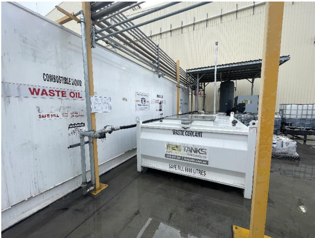
PHOTO 8 Waste oil and waste coolant storage
